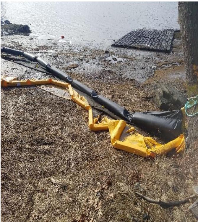
Fig 11: Turbidity barrier in intertidal zone at Gundalow landing/east side of the Bay. Viewing west. (01-27-20).
