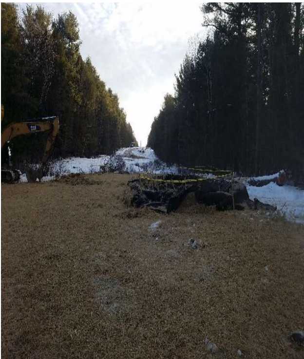
Fig 3: Str. 70 work area and dewatering basin. Viewing east. (01-24-20).
