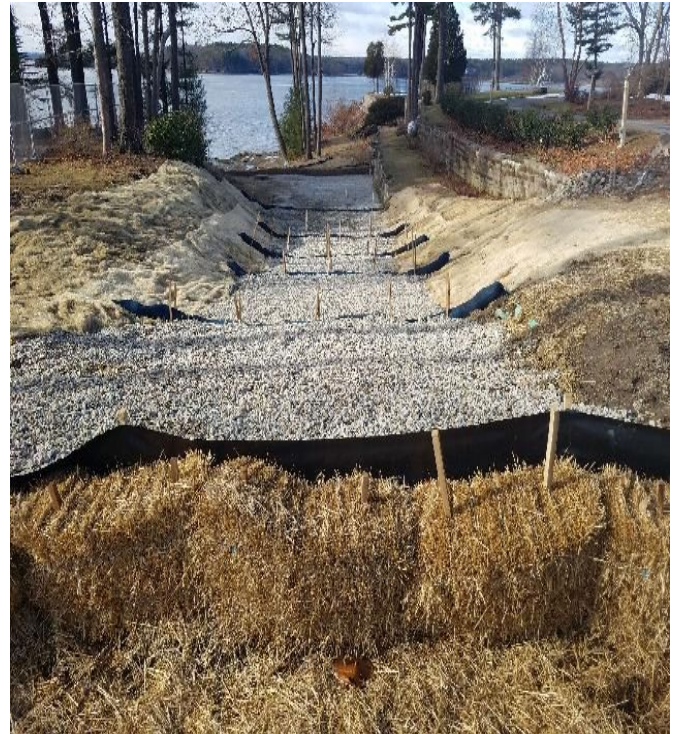
Fig 10: BMPs installed on slope at Gundalow landing/east side of the Bay. Viewing west. (01-27-20).
