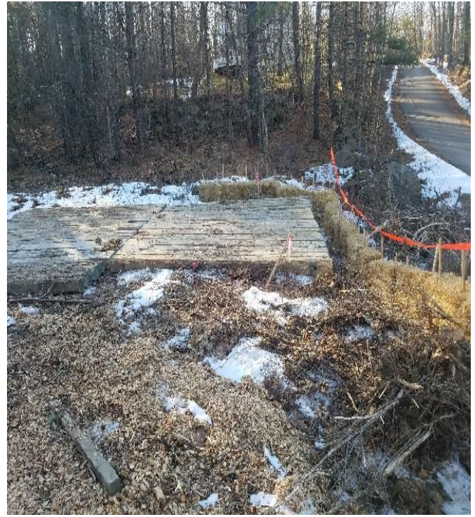
Fig 14: Work pad for Str. 63. Viewing south. (01-29-20).
