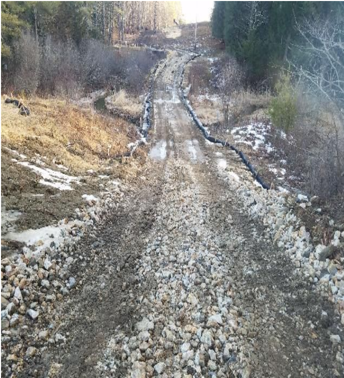
Fig 9 Access road between Strs. 51 and 52. Bridge over stream DS46. Viewing northeast. (01-27-20).
