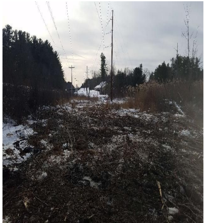
Fig 2: Wetland MW2 after timber mats were removed. Area between Strs. 2 and 3. Viewing south. (01-23-20).
