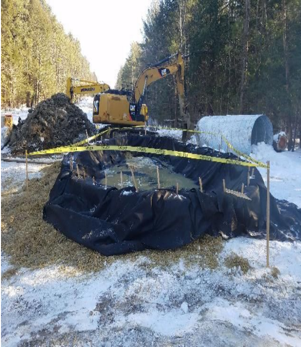
Fig 1: Dewatering basin at Str. 70. Viewing east. (01-23-20).
