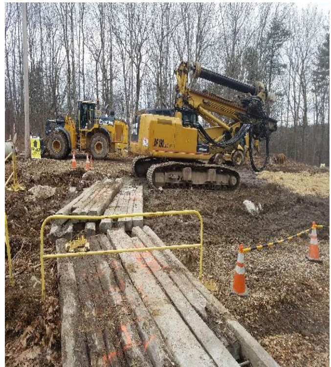
Fig 12: Str. 58 work area. Viewing south. (01-28-20).
