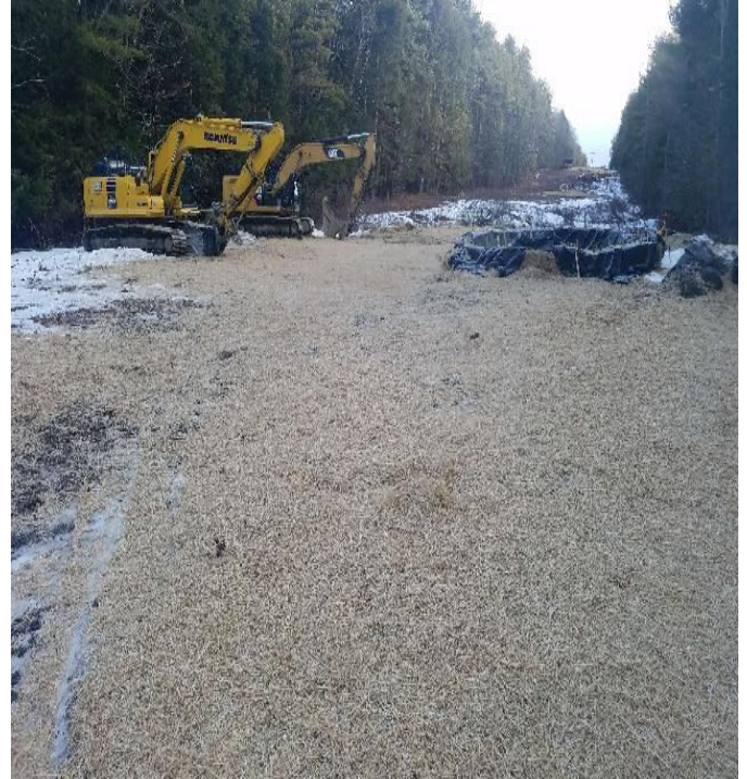
Fig 6: Str. 70 work area. Note straw cover. Viewing east. (01-27-20).
