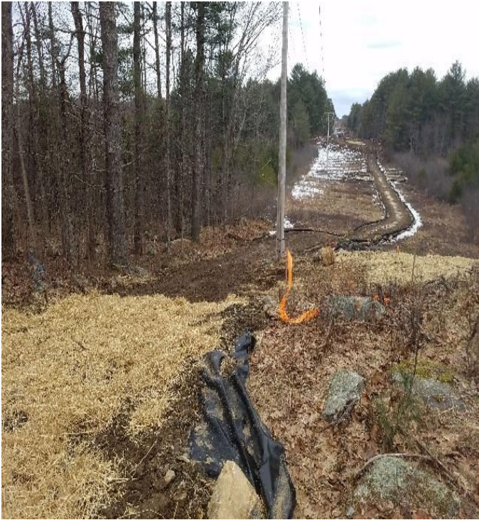
Fig 13: Crew spreading straw over exposed soils leading up to Str. 58. Viewing west. (01-28-20).
