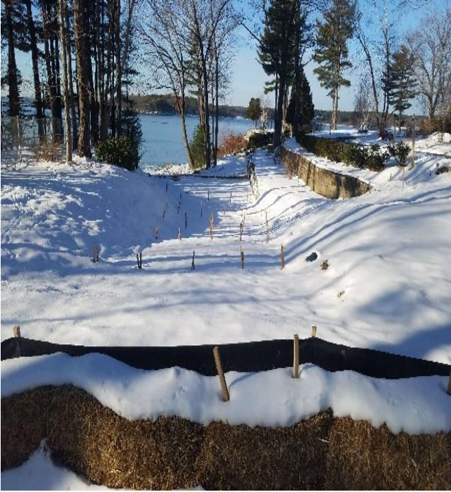
Fig 5: Slope down to vault at Gundalow landing/east side of the Bay. (01-24-20).
